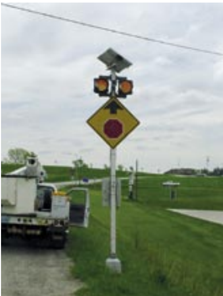
Advance Warning for Stop Ahead
