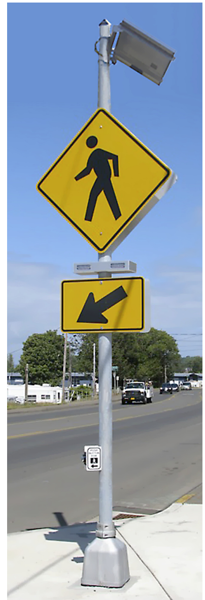
Wrap-around RRFB Light Bar with Required Signage
